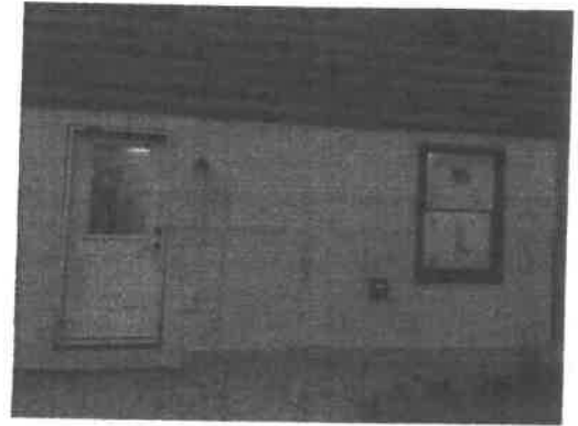
Basement with Door and Egress Window
